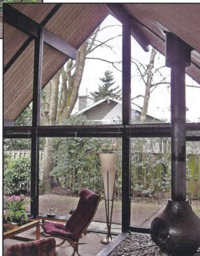
Post-and-beam construction allows walls to be built of floor-to-ceiling glass. Rummer living rooms always faced the rear garden.
