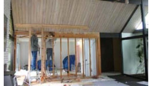
First step was to build temporary shoring to support the roof structure while the beam was removed. This was done for the gable portion in the living room and the flat roof over the master bedroom. With the roof temporarily supported, the portion of the beam to be replaced was cut into sections using a reciprocating saw.
